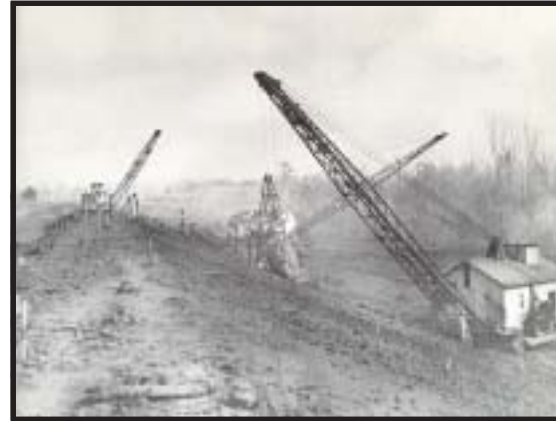
Early levee construction
